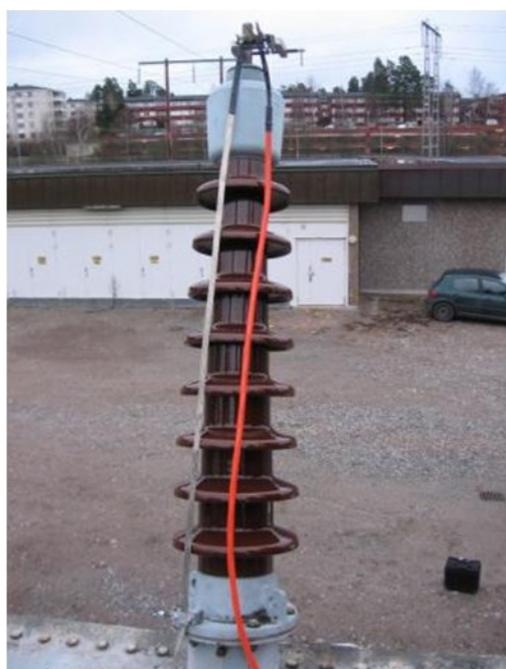
The ground braid shall go from the C-clamp the shortest way to the bottom of the bushing. Good ground connection is essential for reliable test results. Look at the next two pages for more information.
