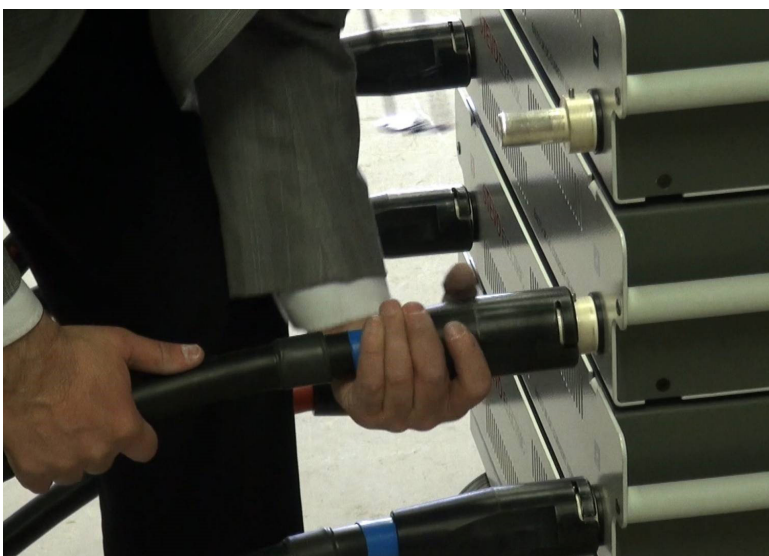
Fig 29: Power cables wiring.
